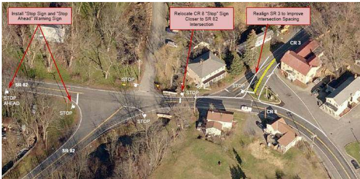
Figure 4: SR 82-CR 3-CR 8 Intersection in Ancramdale
